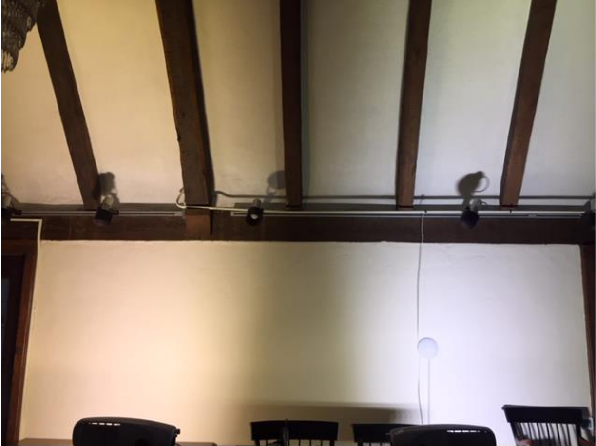
Village of Cayuga Heights LED Street Light Samples. 3000 K on the left and 4000 K on the right.
