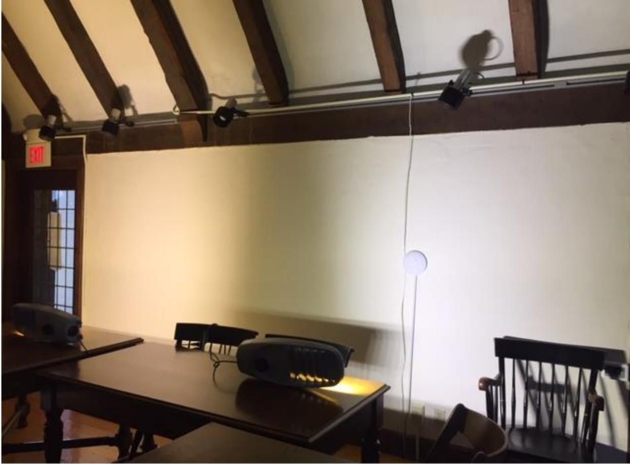
Village of Cayuga Heights LED Street Light Samples. 3000 K on the left and 4000 K on the right.
