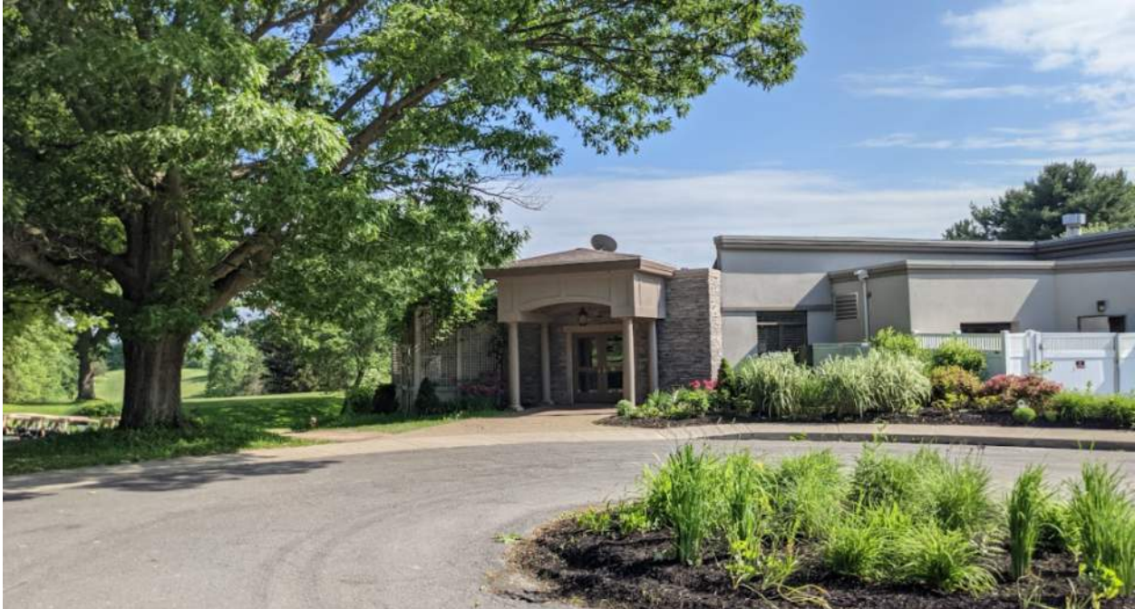
Northeast entrance to clubhouse
