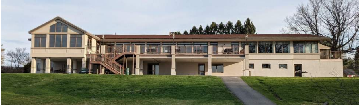
Southside of existing Clubhouse
