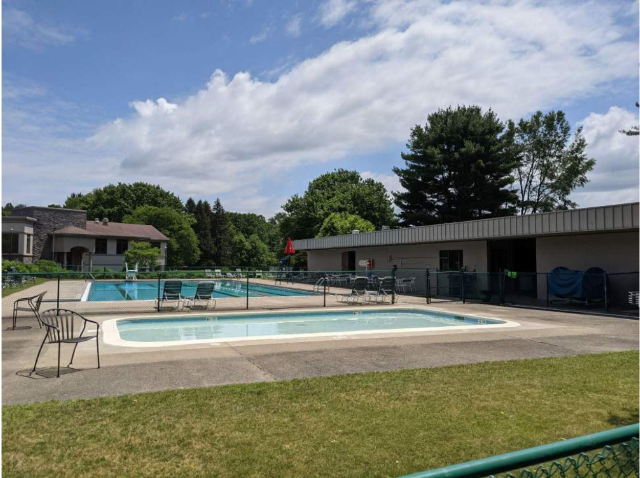
Existing pool and pool house at location of proposed hotel with clubhouse in background.
