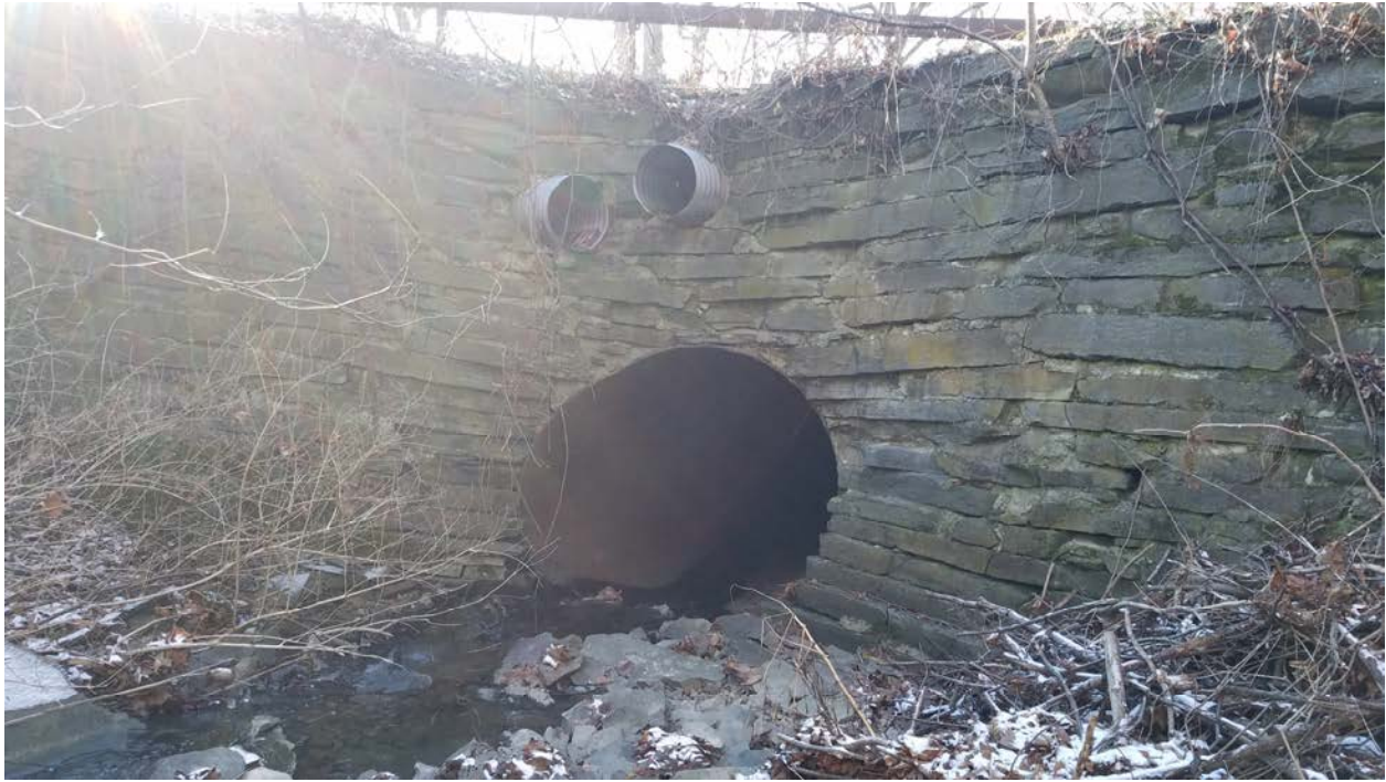
Photo #1 – Inlet side with laid up stone headwall
