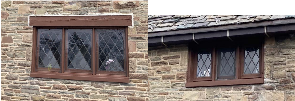
Easternmost windows on Section A's southwest elevation.
