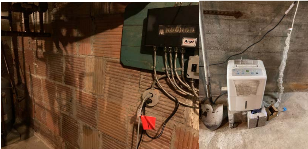
Exposed hollow clay tiles in the basement (L), dehumidifier (R).
