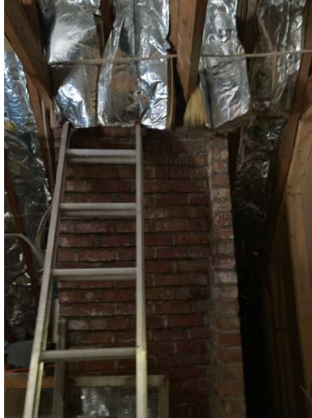
The center chimney of the attic.
